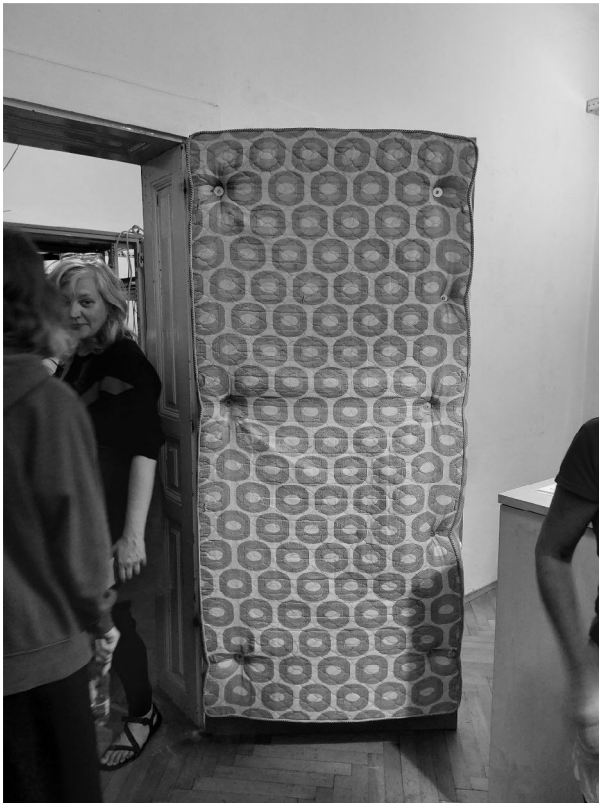
The sound proofing mattress door.
